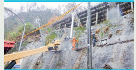
3. Installation of the post
