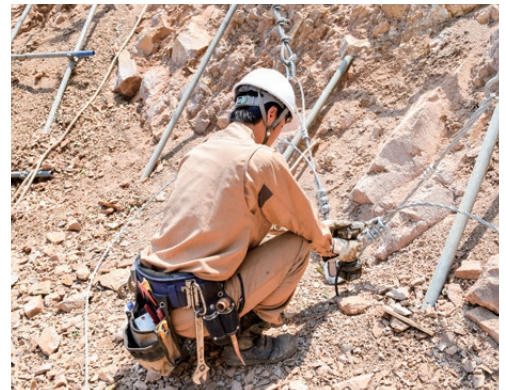
Installing the energy dissipator
