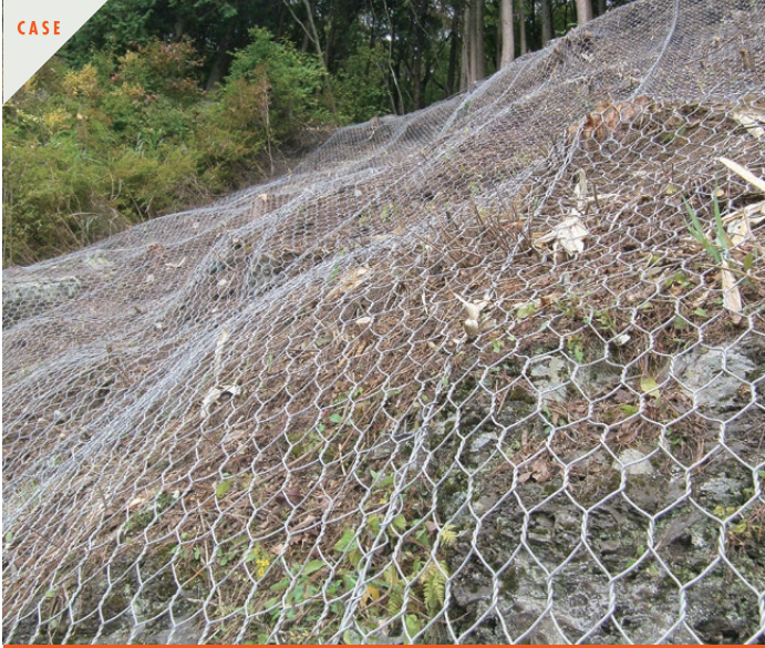
Draped mesh slope protection
