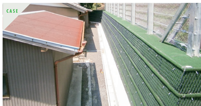
It is possible to install QK Wall in a confined space behind a private house.
