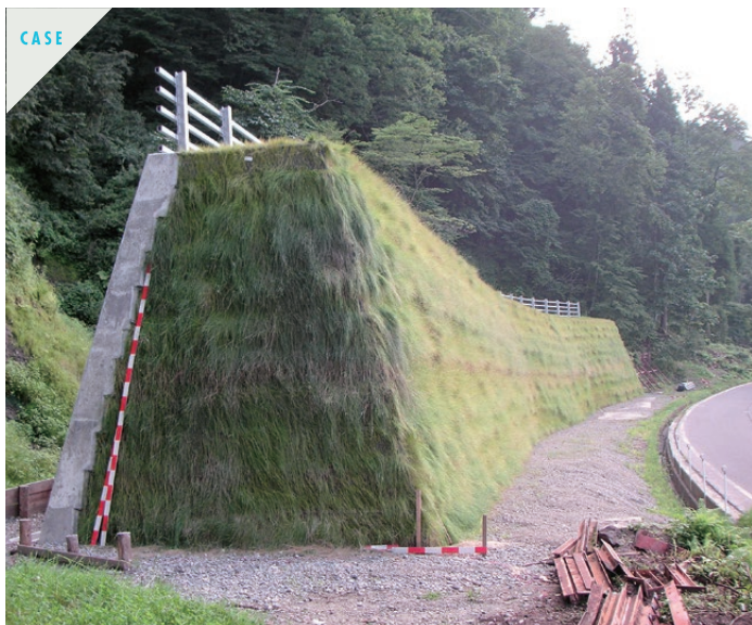
Geo Snow Wall is effective to a location site where a sufficient space is available on the roadside.
