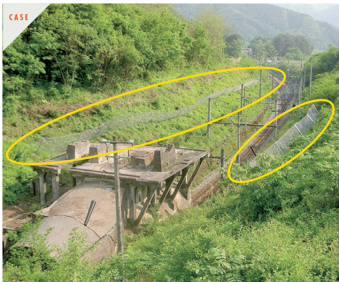
ARC Fences is also effective as the rockfall protection along a railway.
