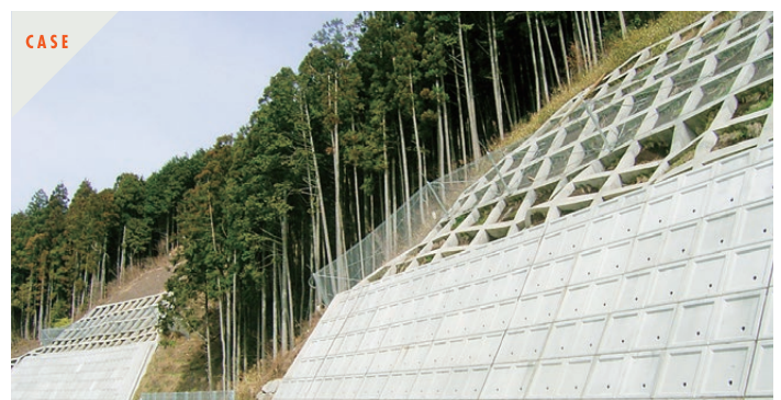
Because the foundation for ARC Fence is the anchors, it can be installed on a slope face on which the frame works are constructed.
