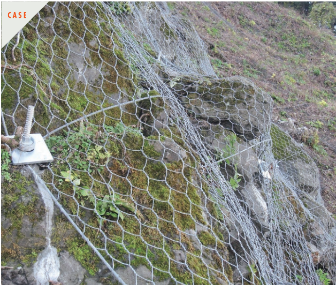
Stabilization of rock slope
