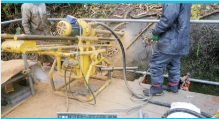
1. Anchor drilling
