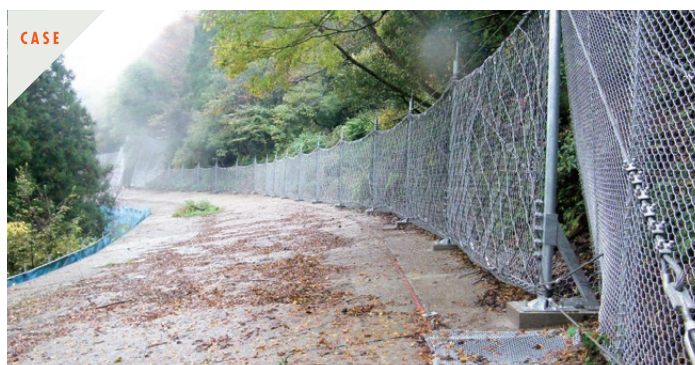
Example of installing SPARC Fence on the snow shed
