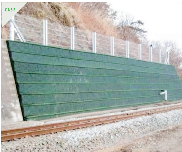
An example where QK Wall was installed adjacent to the concrete barrier by the railway.
