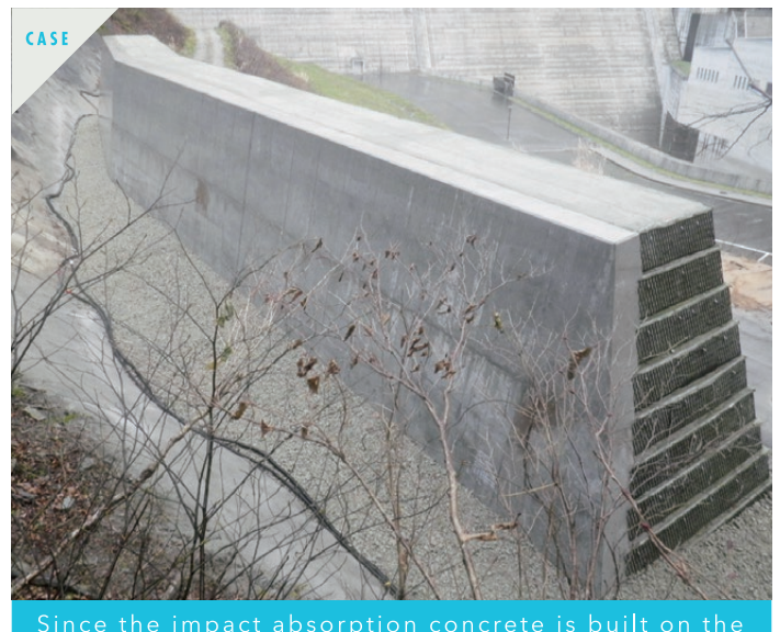
Since the impact absorption concrete is built on the mountainside, the pressure of the deposited snow can be distributed evenly over the impact resistant wall.
