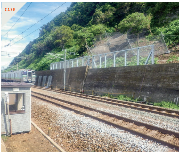
Example where SPARC Fence was installed along the railway
