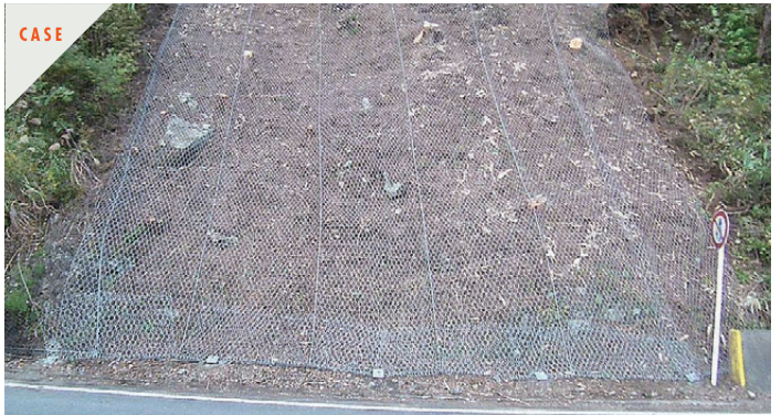
Draped mesh slope protection
