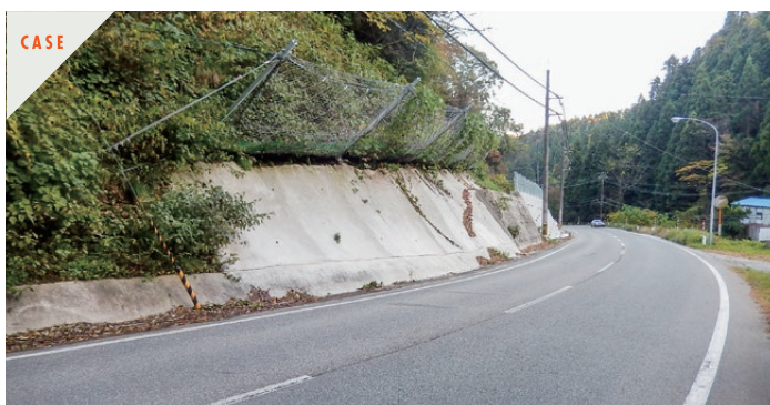
Because the amount of net deformation is small when it catches falling rocks, it can be installed by the road with confidence.
