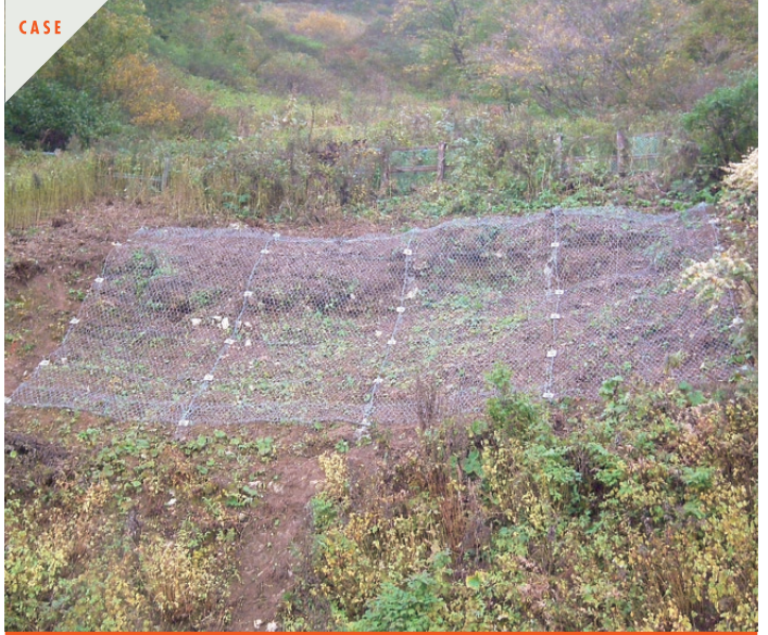
Stabilization of rock slope
