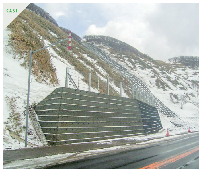
QK Wall can be installed in a confined space on the roadside.
