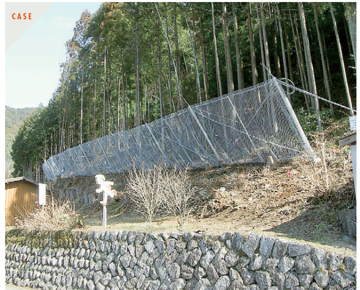
ARC Fence can be installed as close to the object to be protected as possible within the deformation distance of the wire mesh.
