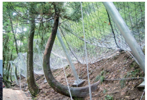
Tra-net Fence can be installed around trees.
